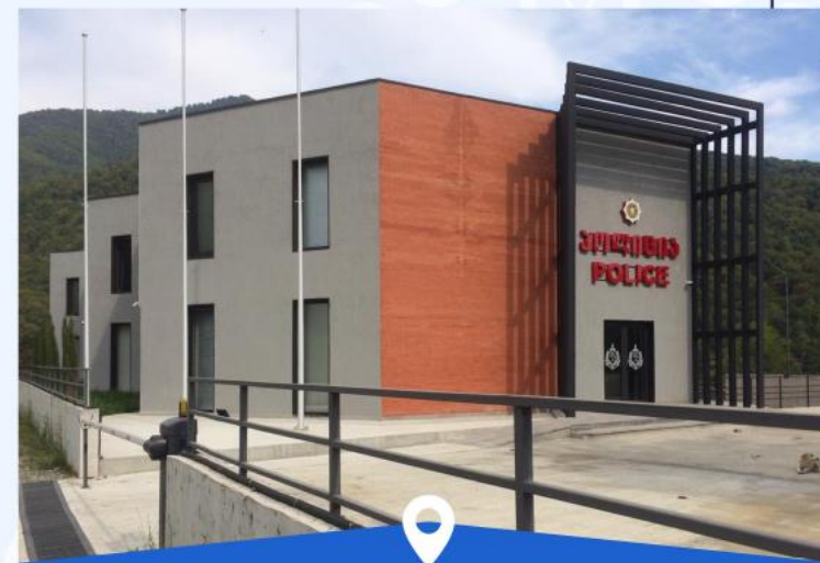
POLICE BUILDING IN DZIBAKHEVI VILLAGE
